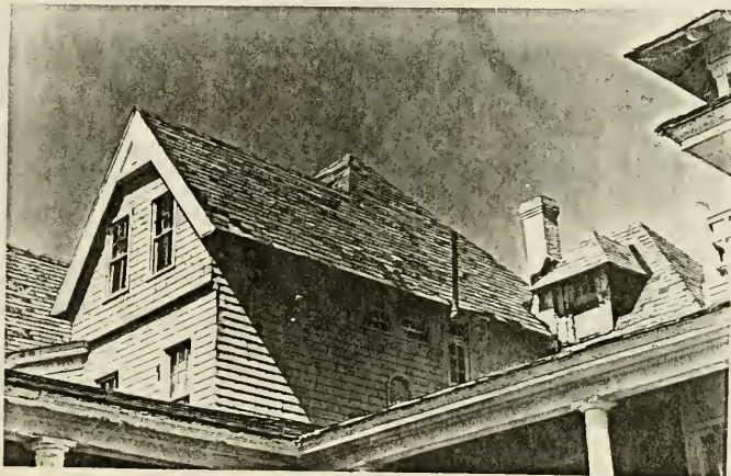
Plate 33: Cottage #2, Roof Area, 1985
